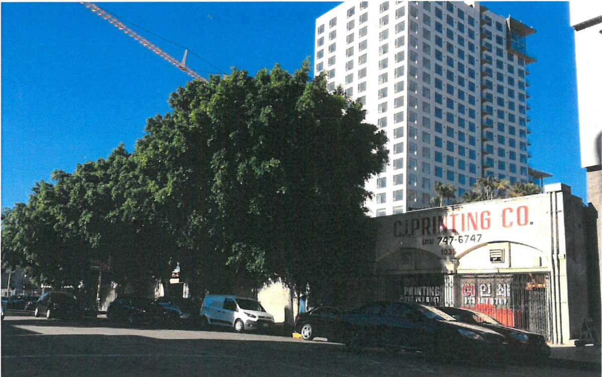
12. Subject site, facing west on Olive St.
