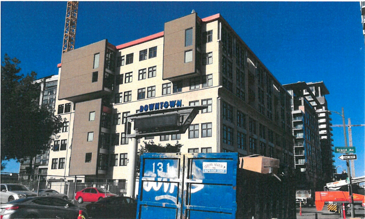
6. Neighboring mixed-use building, facing west on 11 th St.
