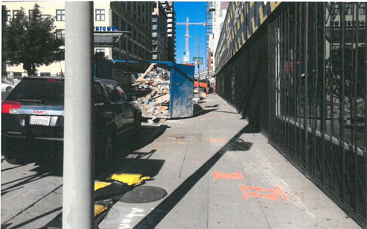
8. Condition of abutting sidewalk on 11 th St., facing northwest.
